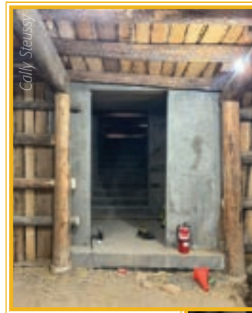
New stairwell out the back of the root cellar
