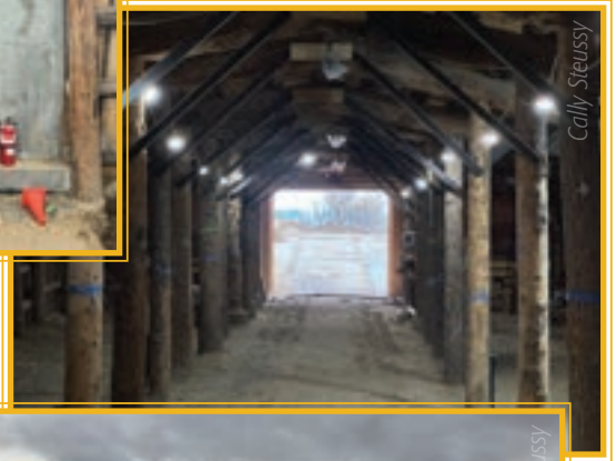
Stabilizing brackets and a glimpse at the new lights
